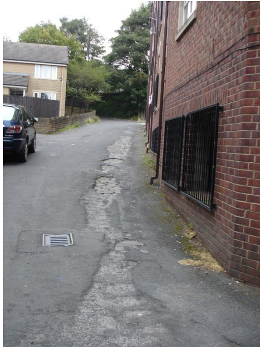
All drain down pipes repaired/replaced
