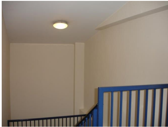
Repaired/replaced lights and emergency lighting
