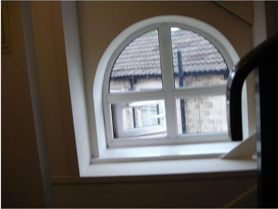
Window openers replaced, (several)
