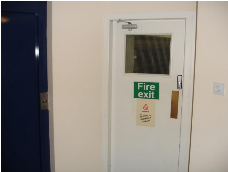
Access to garage from stairwell,
